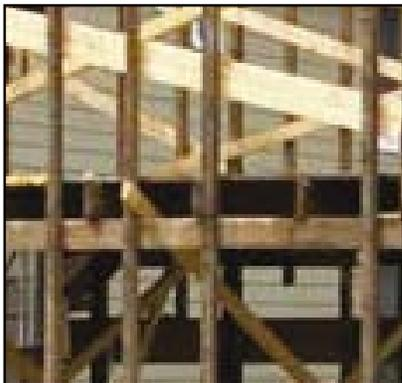
In accordance with the recommendations of the American Forest & Paper Association and building codes, firestopping will be installed in this balloon framing at the ceiling line and floor line.
