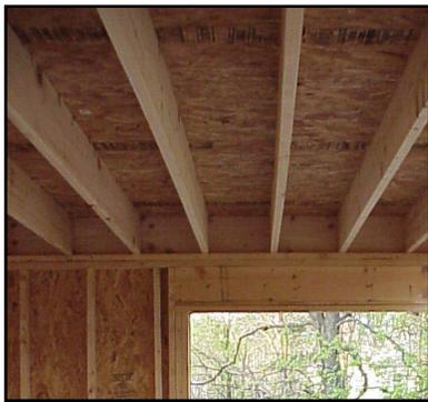
Platform construction provides a structural frame that is fire blocked by virtue of the style of construction—the wall sole plates and top plates isolate the horizontal floor cavity from the vertical wall cavity, as required by building codes. The top plates of the wall prevent movement of fire into the floor cavity. Similarly, the top and sole plates of the wall above prevent fire spread from the floor joist cavity into the walls.
