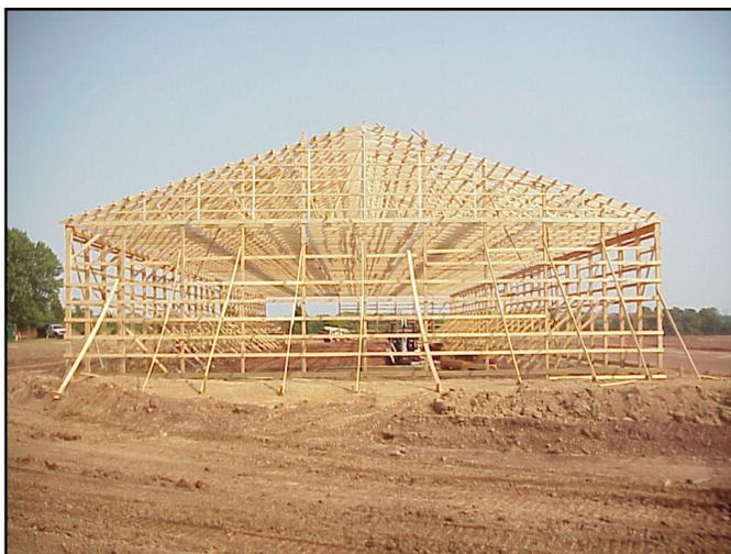
Post frame construction is used widely in the construction of agricultural buildings. Tall columns are embedded in the ground and are braced from buckling by horizontal pur-lins. Roof trusses are supported along the length of the wall by headers attached to the tops of the columns.
