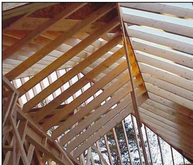
Dimension lumber is used for wall and roof framing. When lumber is used for roof framing, it is referred to as rafters. This complex rafter framing will be extremely difficult to detect once the sheathing and drywall are installed.
