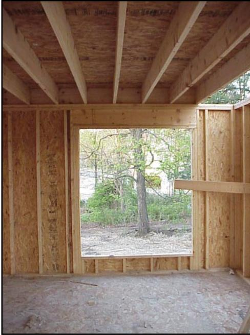
Platform construction is today's most common method of construction. It combines safety for framers while the building is under construction, with inherent firestopping once the walls are sheathed.
