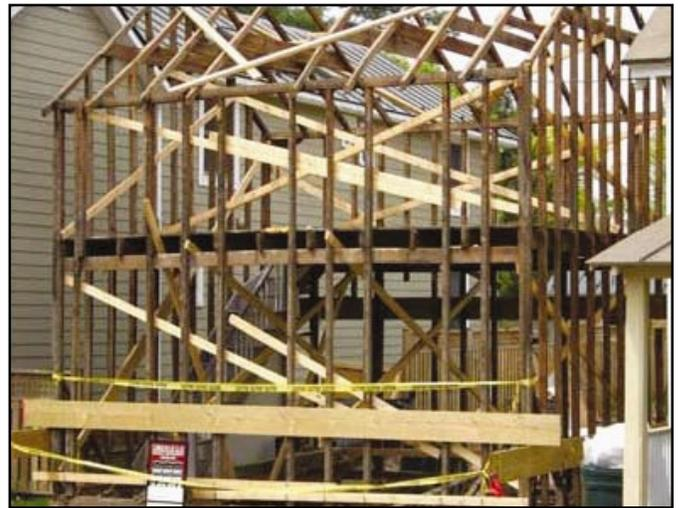
Early house construction was “balloon” framed. This house, undergoing major renovation, is a good example of balloon framing. Unless firestopping is added, fire within the wall can easily spread vertically, since there are no top plates. Fire originating in the floor/ceiling assembly can spread horizontally and eventually vertically through the walls.
