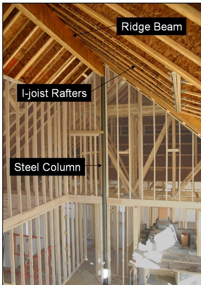
I-joists are used as roof rafters where high, open ceilings are desired, such as this 2<sup>1</sup>/<sub>2</sub>-story room. The I-joists are supported at the ridge by an LVL ridge beam. Since there are no ceiling joists to resist outward thrust, the I-joists must be supported at both ends. The load on the ridge beam is carried by columns to the foundation.
