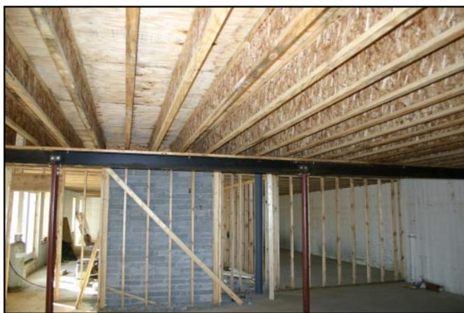
I-joists used in a typical basement floor assembly. In this figure, the I-joist spans from the exterior walls, over a steel beam to an interior bearing wall.
